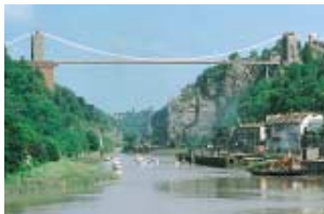
Clifton Suspension Bridge, Bristol.
