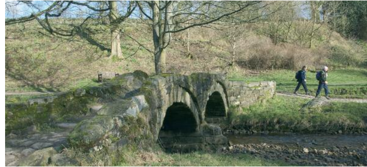
Ancient footbridge, Wycoller
